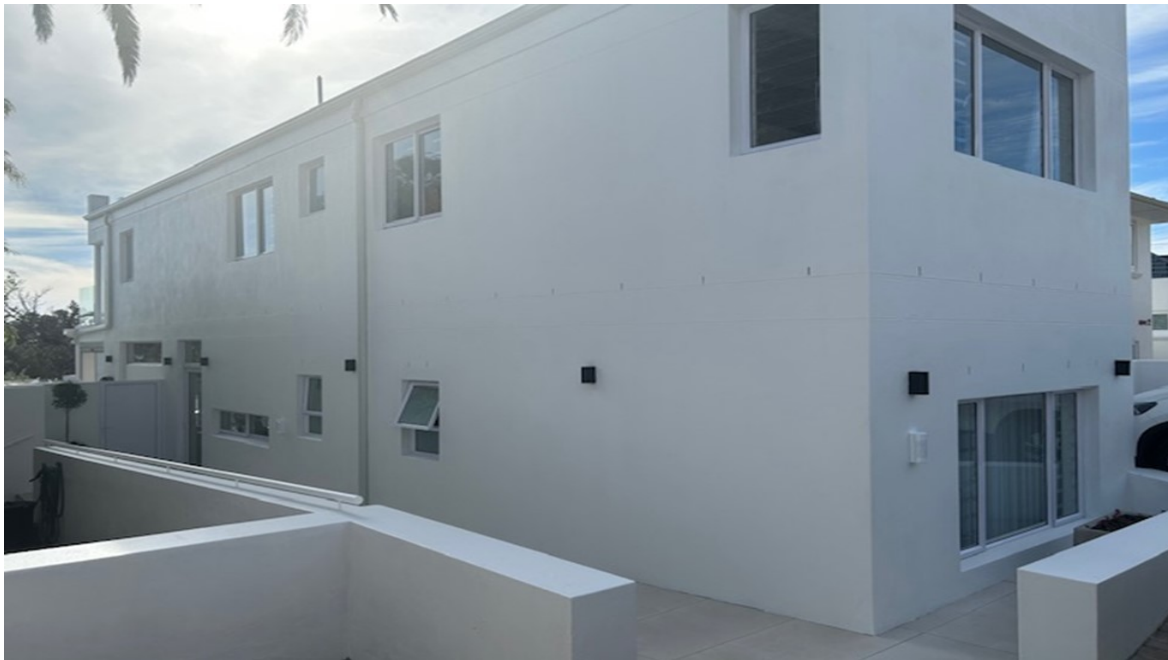
Figure 8: The ground floor of this portion of the building has been converted into a 'second dwelling unit'.
